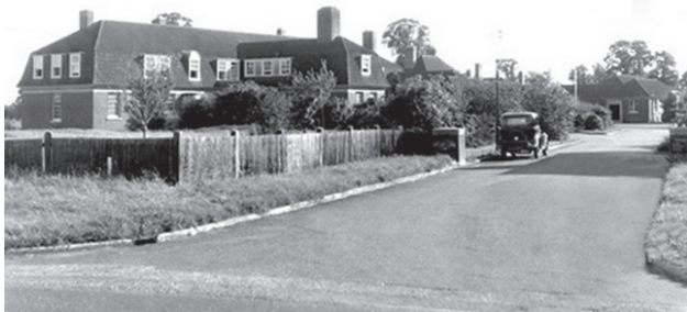
Newly built Melksham Hospital on Spa Road in the 1950s
